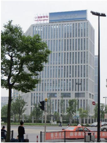
Figure 5. Internet of Things (IoT) Shanghai building, Jiading, Shanghai, China.
